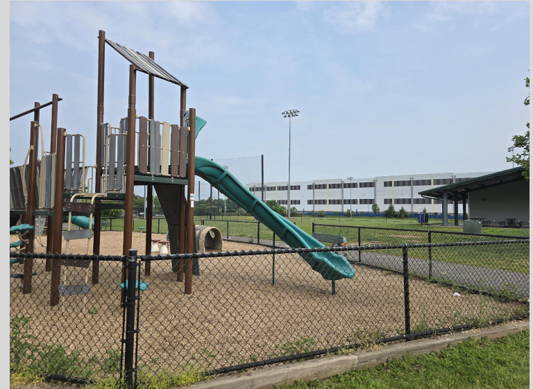
Photo: An Amazon data center (background) next door to a playground (foreground). Credit: Ben Inskeep | CAC
