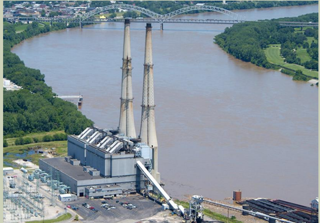
Photo: Coal-fired Gallagher Station, Floyd County, IN, retired in 2021. Credit: Duke Energy.
