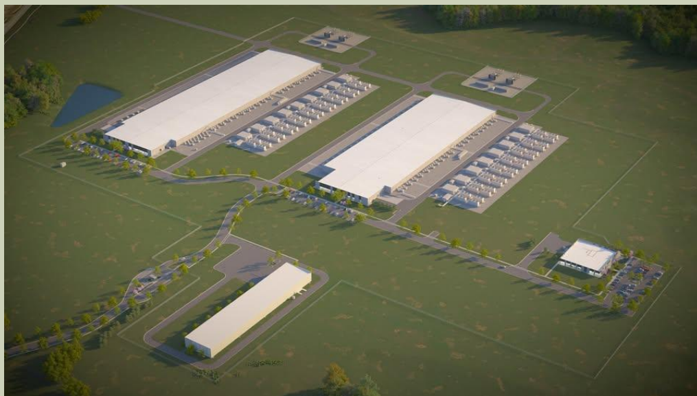
Source: Meta, Jeffersonville Data Center
