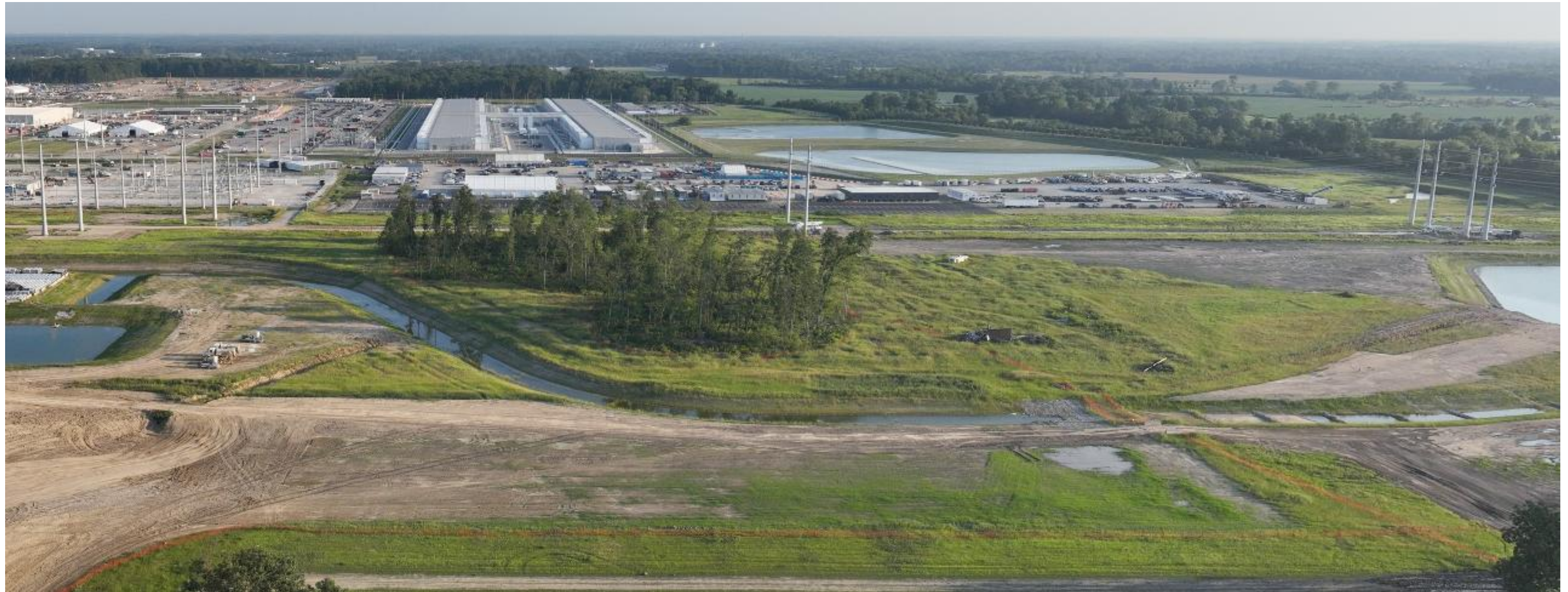
Project Zodiac Phase 3 Permit Area: Wetland 47 (looking north)
